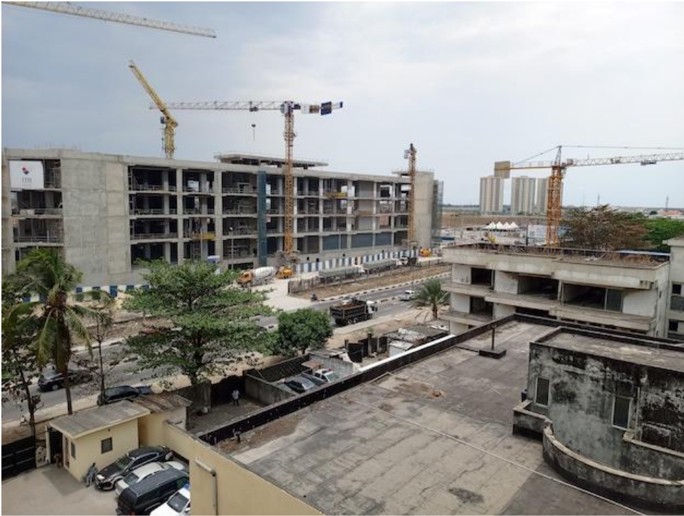
High-rise buildings under construction in Lagos, Nigeria. Most accommodation is unaffordable for young Nigerians. Credit: Promise Eze/IPS
